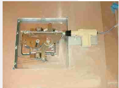
Connect Nylon Rod Connector To Latch
